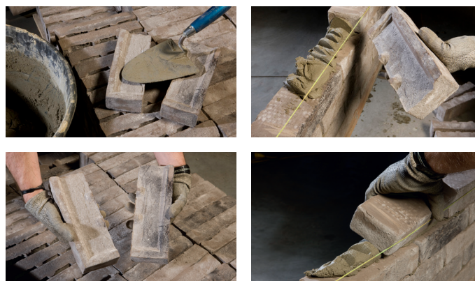
Photo 3: positioning of Iluzo bricks
