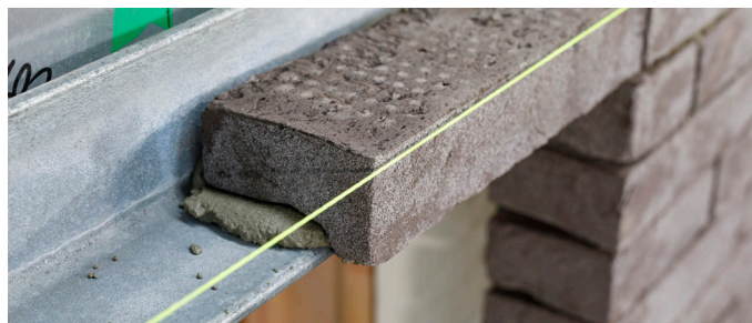
Photo 6: placement of L-profile
