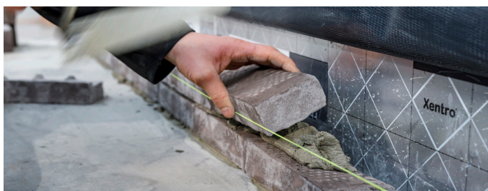
Photo 5: placement of mortar
