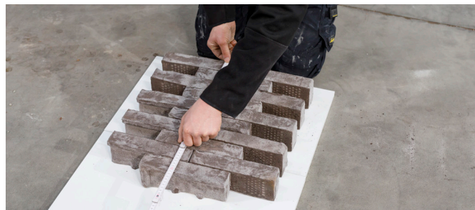
Photo 4: laying out Iluzo bricks
